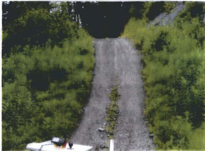
Photo 6. Steep grade between Stations 6 and 7.
