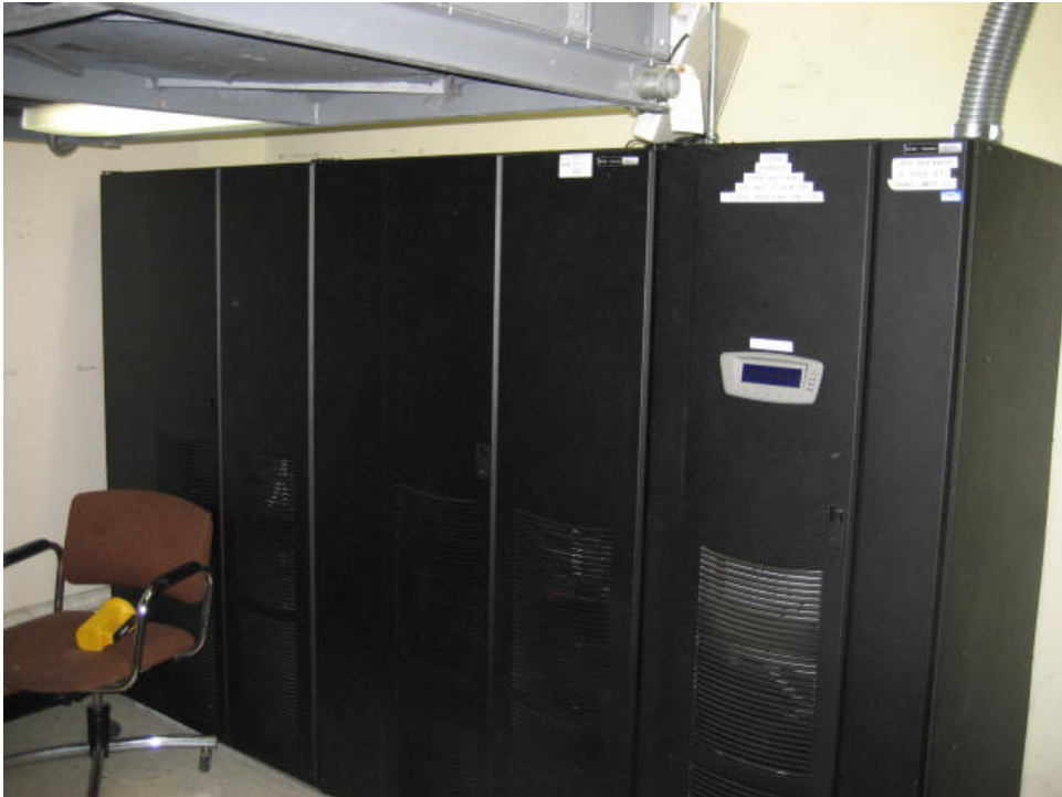
Photo 1: Existing IT Server Room AC Unit
