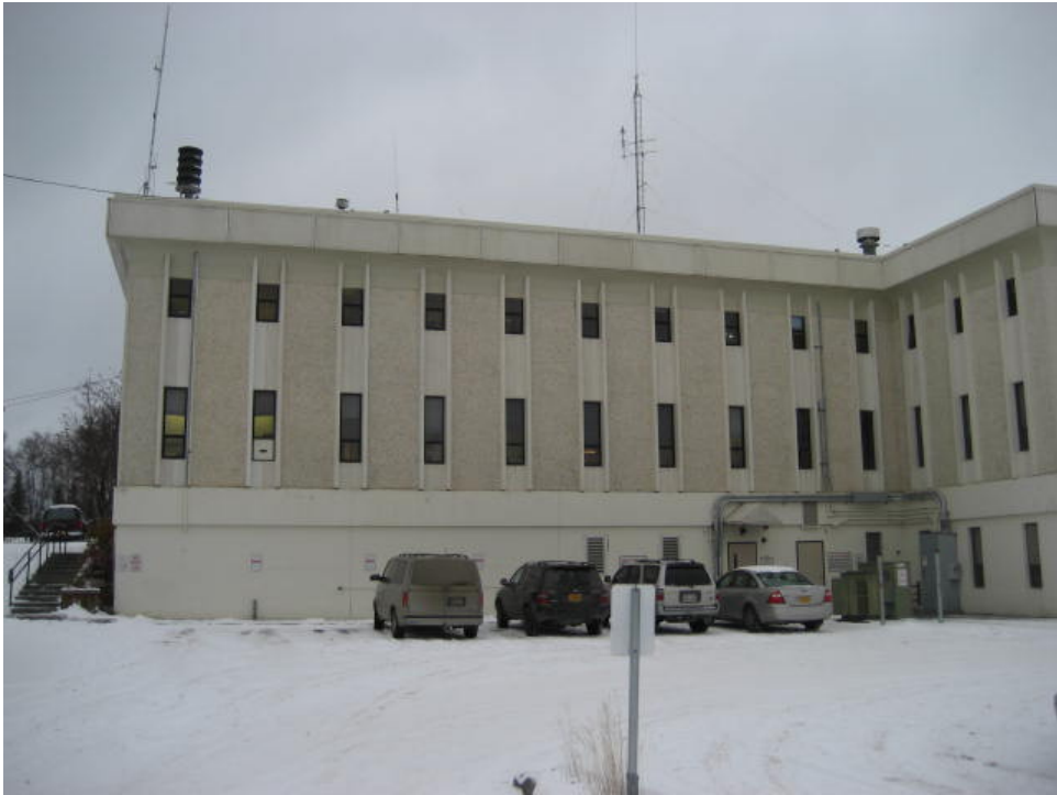
Photo 4: Proposed Location for New Condensing Units on Building Wall
