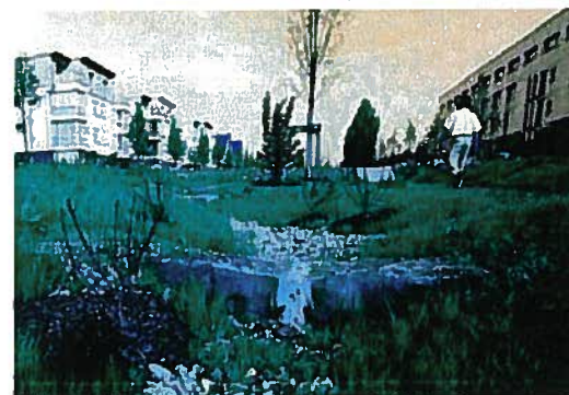
Planted bioswale near trail conveys stormwater.
