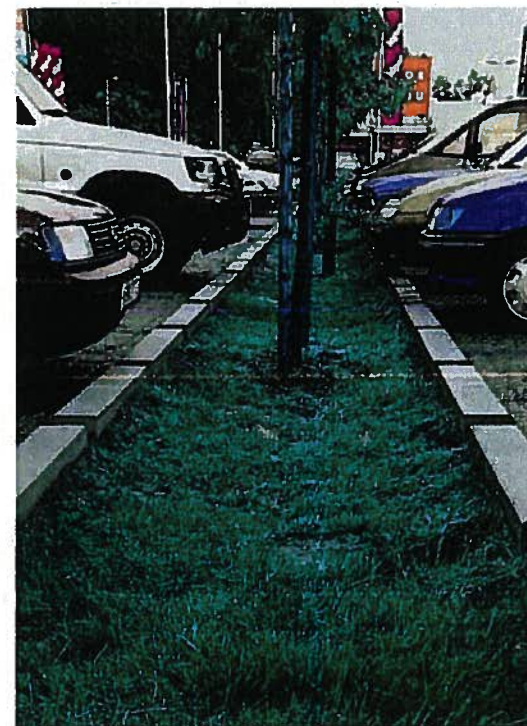
Planted swale separates parking stalls and collects stormwater.
