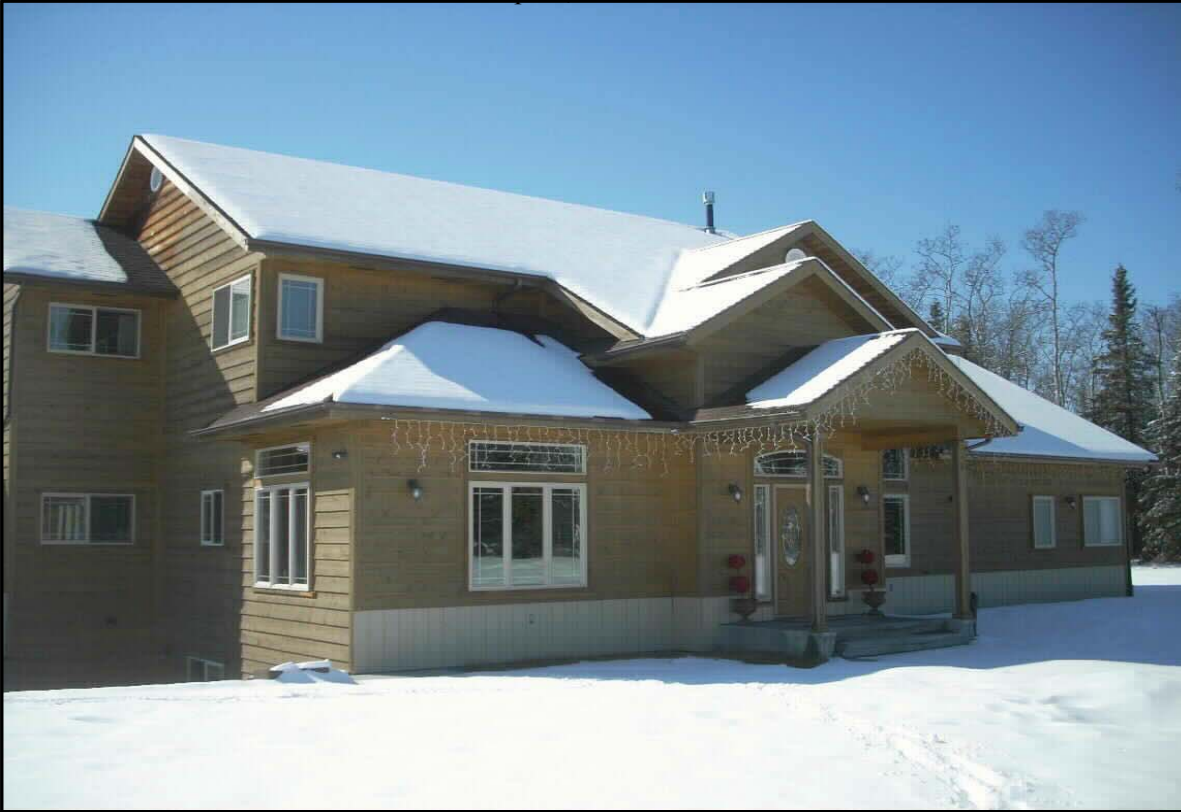
FRONT VIEW OF SUBJECT PROPERTY
