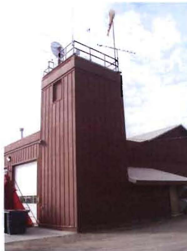
Pic #2 South-east View
