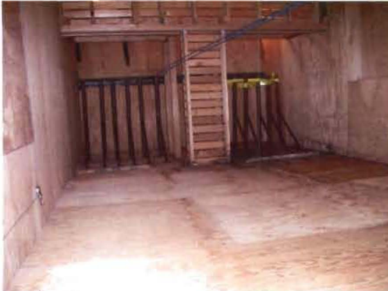
Pic #3 View up tower East Side
